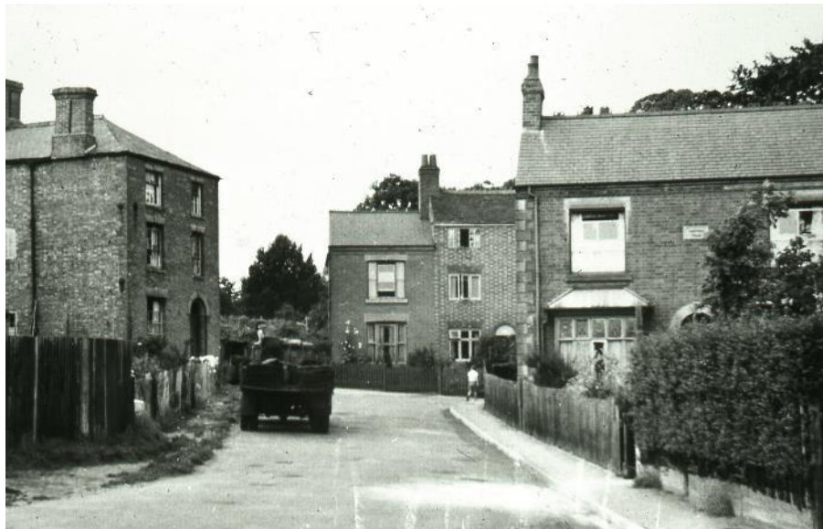
Obenbach House, Church Street
