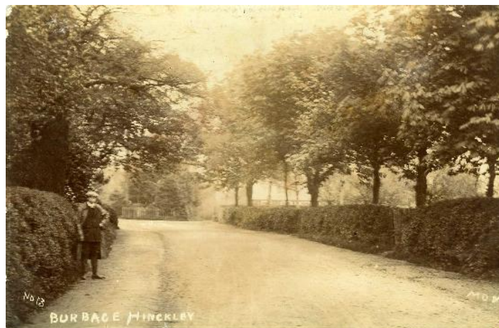
Location of Burbage Experimental Station, Grove Road
