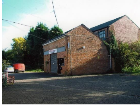
Previously the Coop Bakery, Church St
